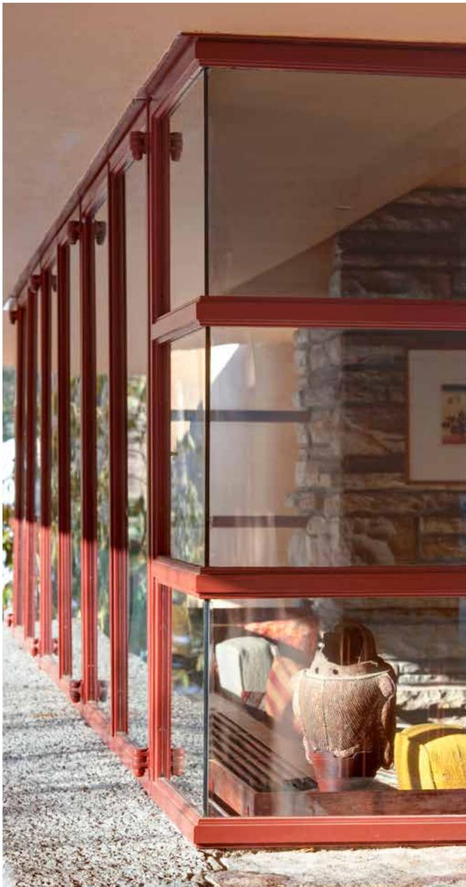
*The superior edge performance of SentryGlas® meant that the architect could use a butt-joint design where the panels met.*
