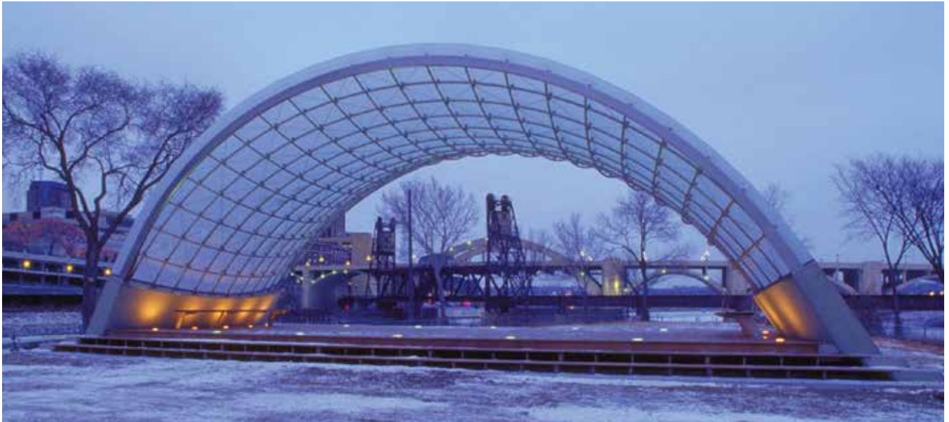
The sculpted shape of the bandshell is designed to let the mighty Mississippi River flow right through during flood stages.
