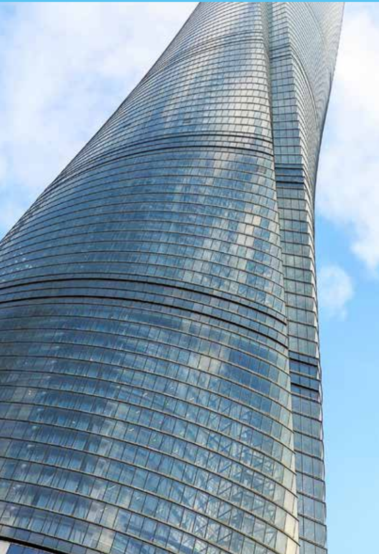
The Shanghai Tower takes the form of nine cylindrical buildings stacked atop one another, all enclosed by the inner layer of the glass façade, which completes a 120-degree twist as it rises. This design reduces wind loads on the building by 24%.
