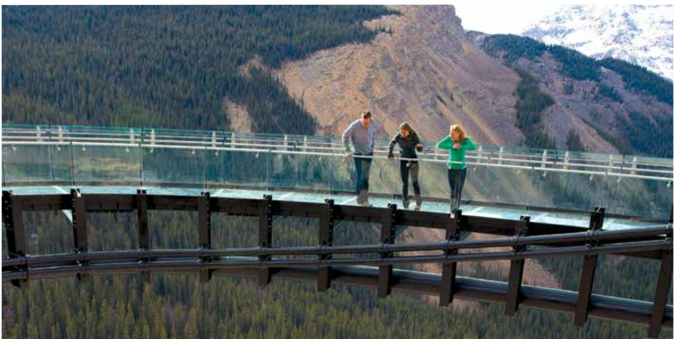
The breathtaking Glacier Skywalk, jutting out from the cliff face, is a superb example of SentryGlas® ionoplast interlayers in action.
