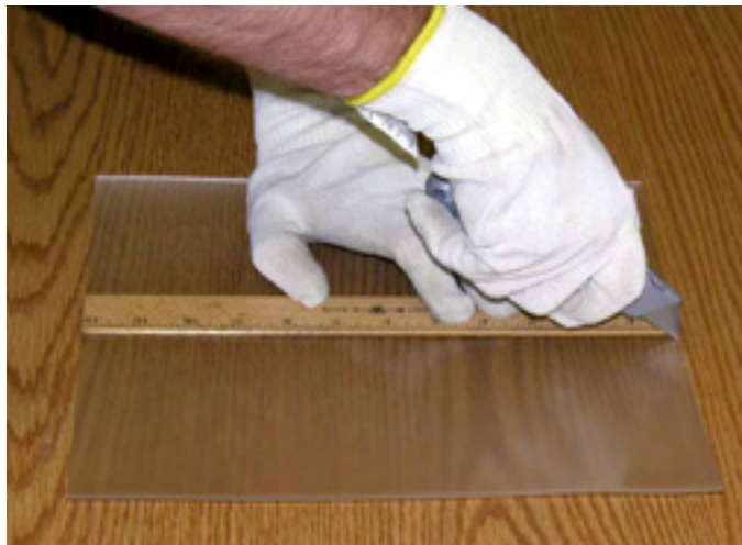
FIG 9 • Cutting SentryGlas®: Score pattern using a utility knife
